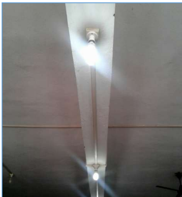
Photo 5 and 6: Ordinary fluorescent lamps are replaced by CFL in passages
