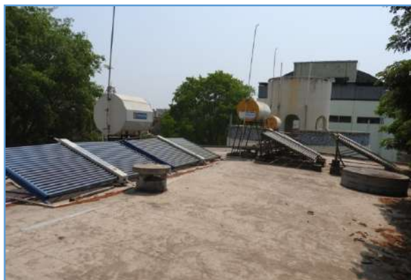
Photo 7- Solar water plant on roof for hot water requirement
